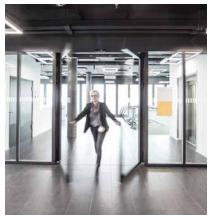
**In day-to-day use** smoke and fire-rated automatic sliding doors offer the convenient advantages of automatic doors: contactless, barrier-free access.
